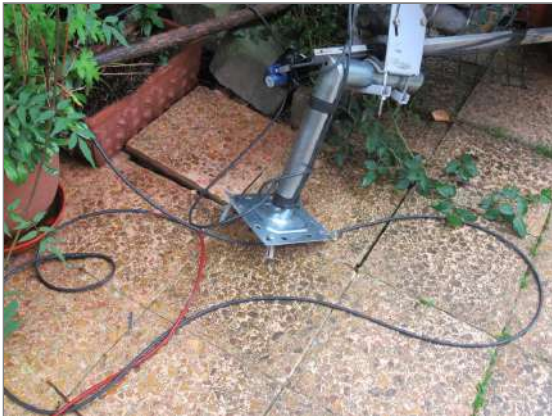
Photo - 150 Paving slabs were noted to be loose on the rear pathway
