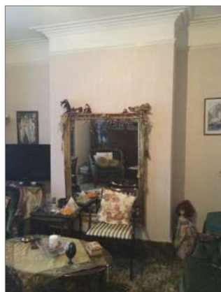
Photo - 105 Chimney breast in front living room
