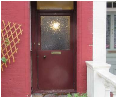
Photo - 49 Front door
