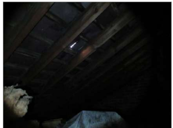
Photo - 65 Gaps were noted to the roof covering
