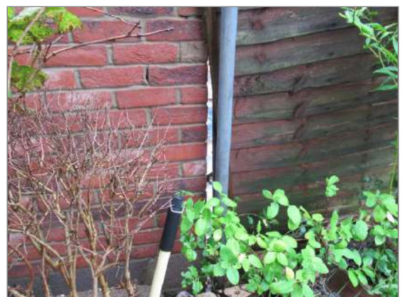
Photo - 147 The rear left-hand boundary fence was noted to be defective
