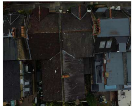
Photo - 11 Main roof as viewed from above
