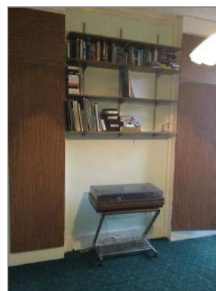
Photo - 108 Chimney breast in first left hand bedroom
