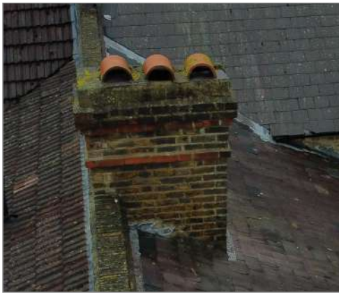
Photo - 6 Right-hand chimney stack side view
