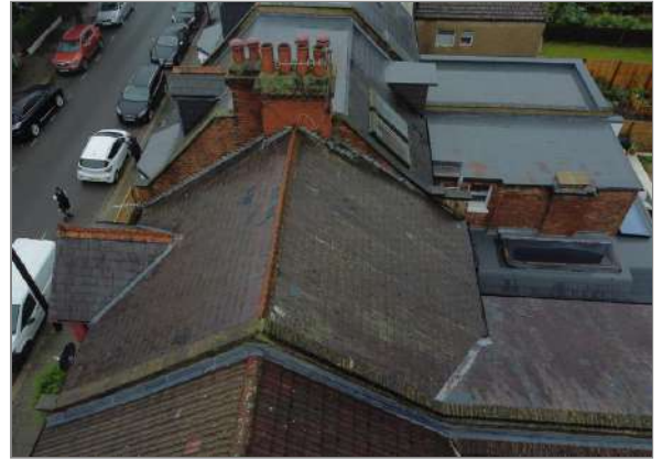
Photo - 9 Main roof side elevation
