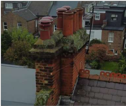
Photo - 2 Left-hand chimney stack
