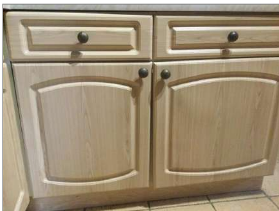
Photo - 111 The cupboard doors were noted to have dropped on their hinges
