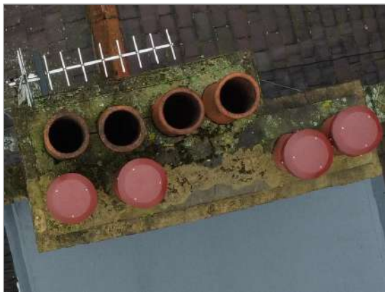
Photo - 4 Left-hand chimney stack as viewed from above
