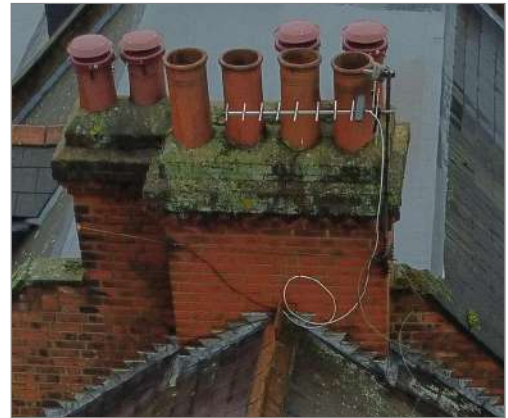
Photo - 3 Left-hand chimney stack side view
