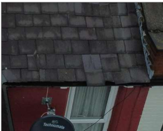
Photo - 23 A slipped tile was blocking the guttering on the front elevation
