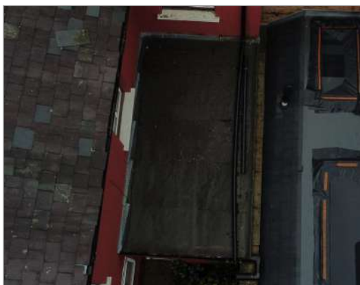
Photo - 20 Flat roof to the rear of the property
