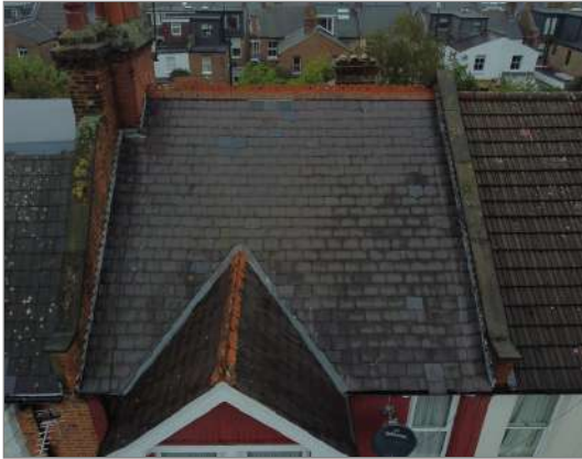
Photo - 8 Main roof front elevation
