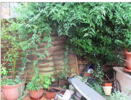
Photo - 146 The rear left-hand boundary fence was noted to be defective
