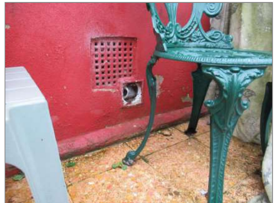
Photo - 38 An uncovered vent was noted to the rear elevation wall
