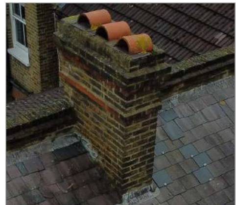
Photo - 5 Right-hand chimney stack
