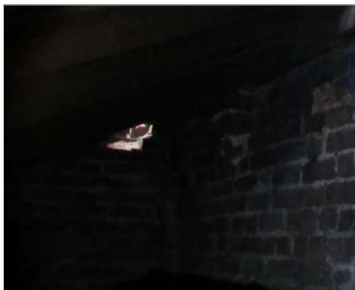
Photo - 68 A hole was noted to the wall in the roof space
