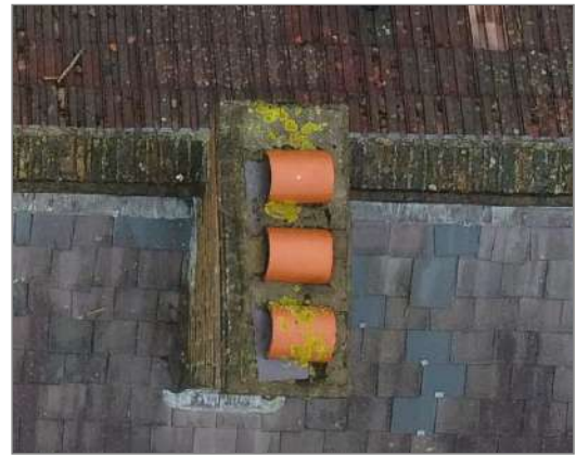
Photo - 7 Right-hand chimney stack as viewed from above
