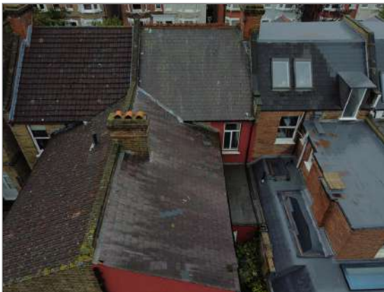
Photo - 10 Main roof rear elevation
